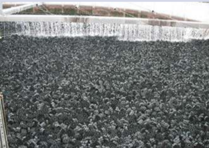
The plastic media inside the bio-trickle tanks.
