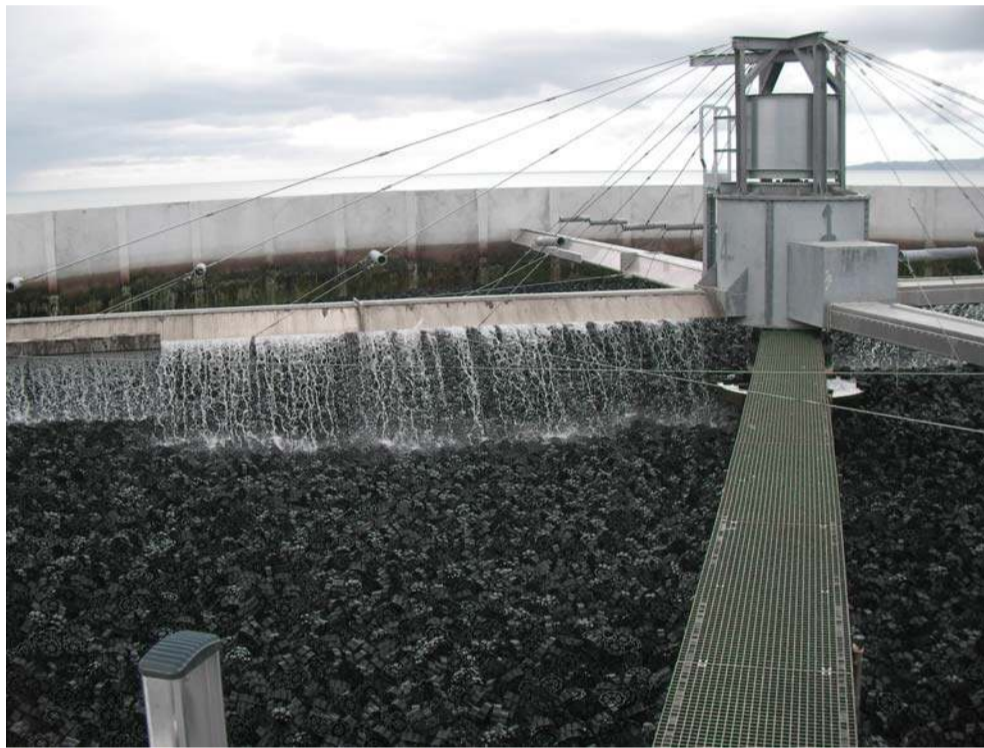
The bio trickling filter tanks in operation at the wastewater plant in East Clive.
