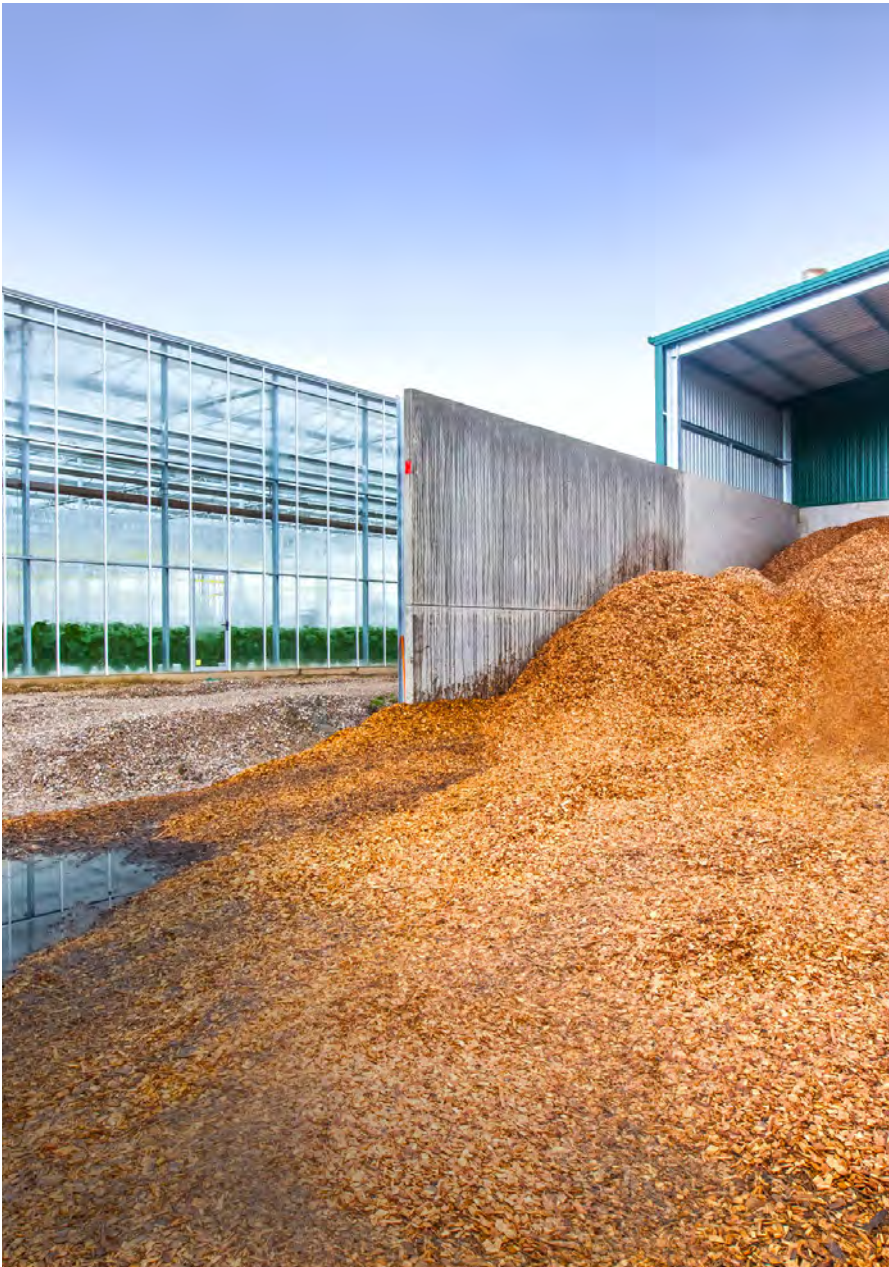
Prize-winning glasshouse at K&L Nurseries near Christchurch burns green waste, eliminating 3,500 tonnes of CO2 emission
