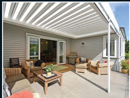
A translucent opening roof allows natural light in even when fully closed
