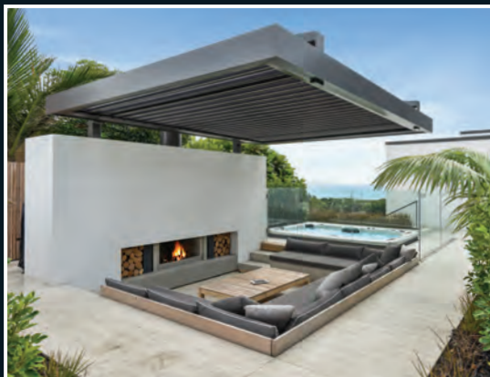
Custom designed opening roof and frame suspended below steel supports
